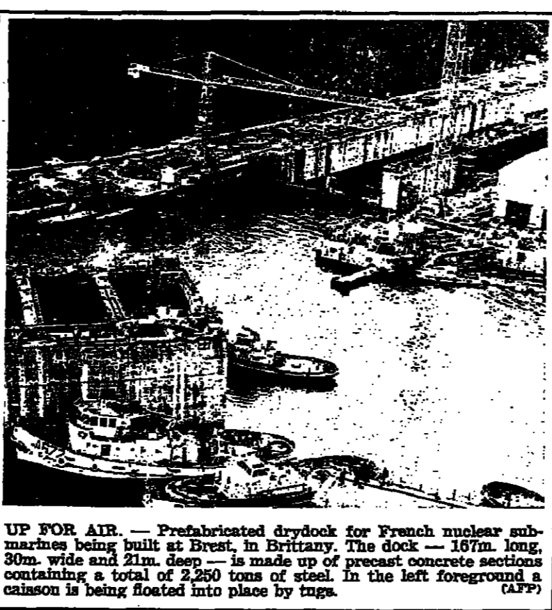
UP FOR AIR. — Prefabricated drydock for French nuclear submarines being built at Brest, Brittany. The dock — 187m long, 30m wide and 21m deep — is made up of precast concrete sections containing a total of 2,250 tons of steel. In the left foreground a caisson is being floated into place by tugs.
